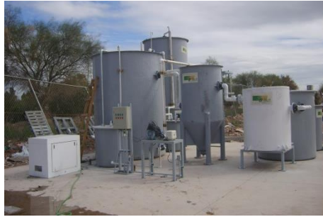
Package Plant for domestic water with a capacity of up to 100 m 3 /d (IBPak®)
