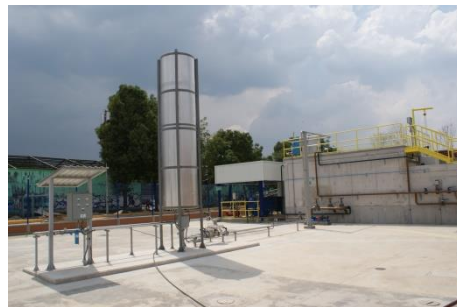
Biogas burner
