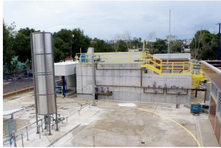
WWTP general view
