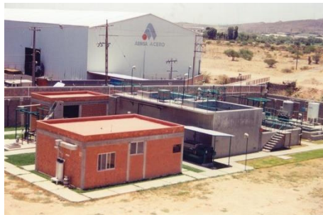
WWTP general view
