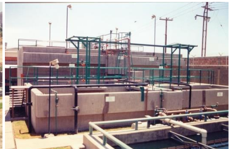
WWTP general view
