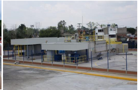
WWTP general view
