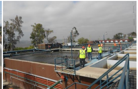
Evaluation of the physical conditions of 234 WWTPs with capacity less than 100L/s
